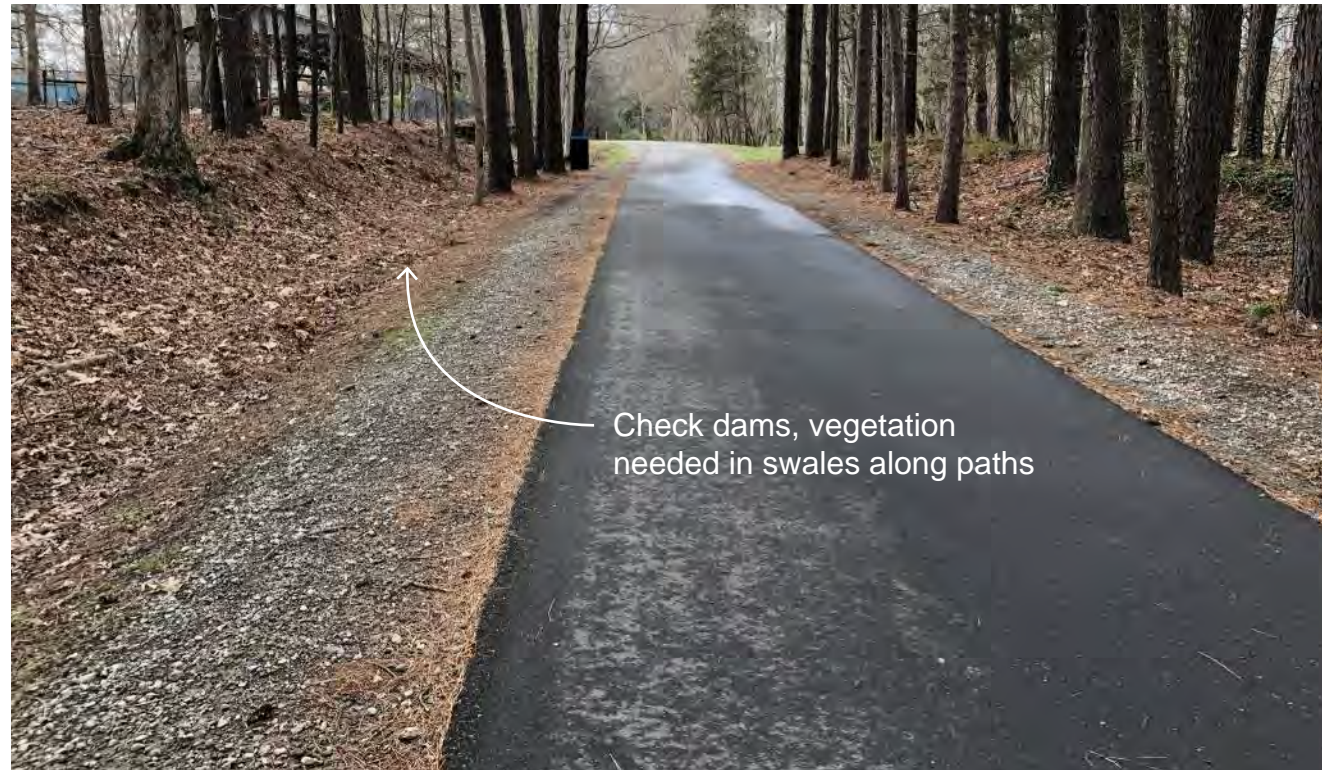
Existing swale along path; Photo: Andropogon
