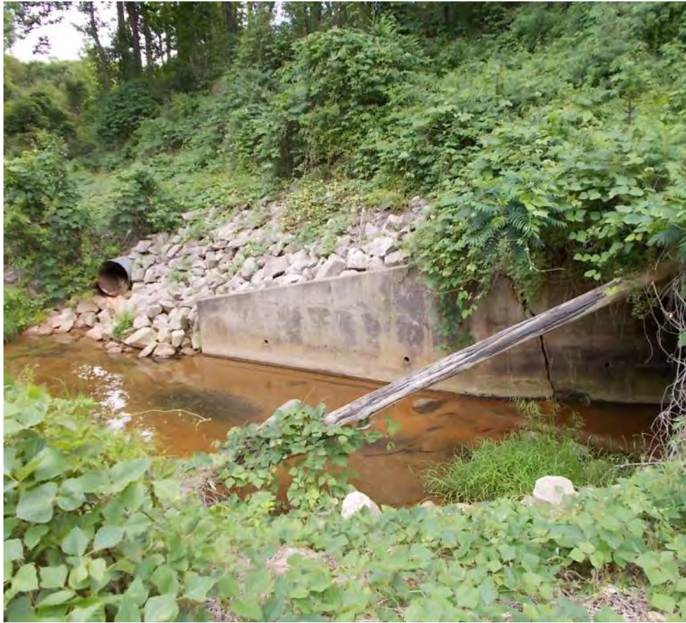
House Creek entering the NCMA from Wade Ave culvert (May)
