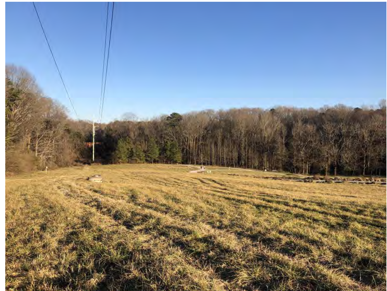
Existing power lines through Lower Meadow, looking toward I-440; Photo: Andropogon
