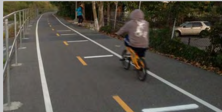
Figure 12. Rumble Strips on L.A.'s Riverwalk Bike Path
