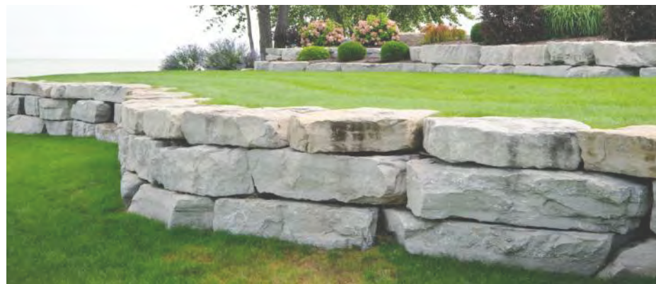
Examples of terraced rough-cut stone retaining walls; Photos: Andropogon (top) and Esch Landscaping (bottom)
