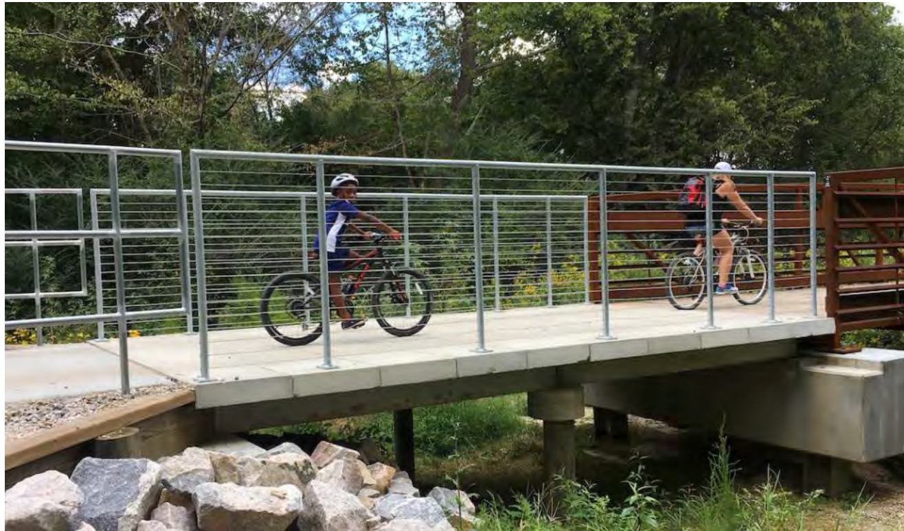
Bridge spanning the entire floodplain, Sanford Creek Greenway, Wake Forest, NC; Photo: PermaTrak
