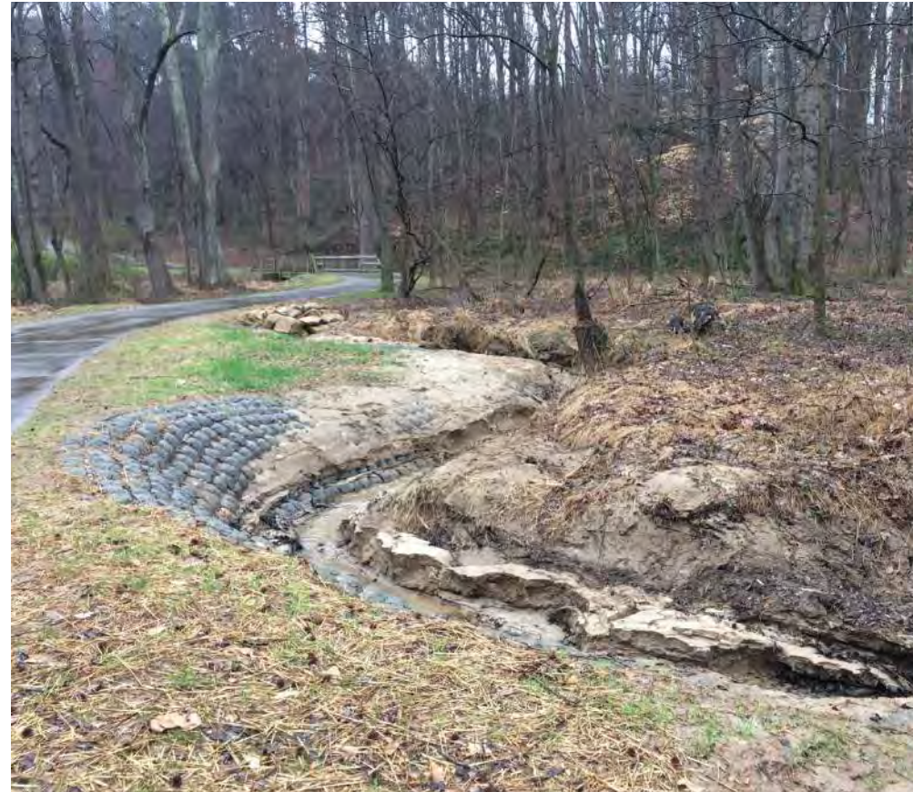
Bank reinforcement at greenway trail (February)
