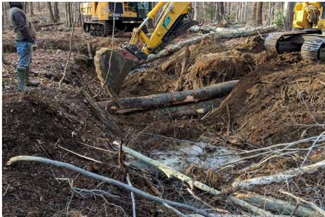
Construction: installation of log check dams
