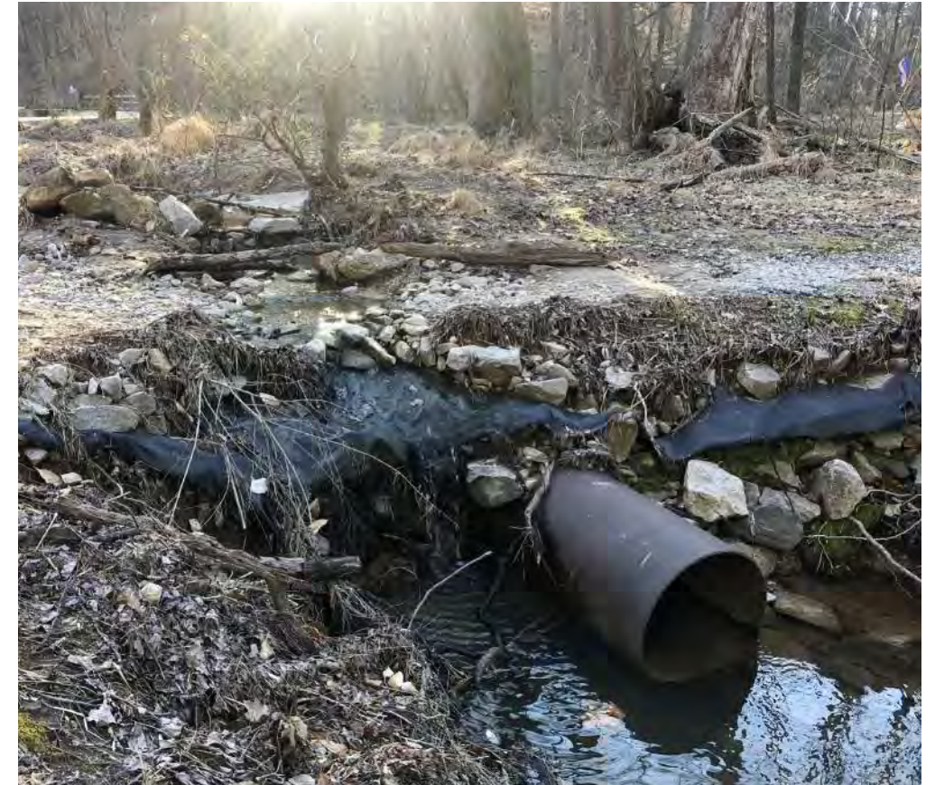
Buried culvert near confluence (February)
