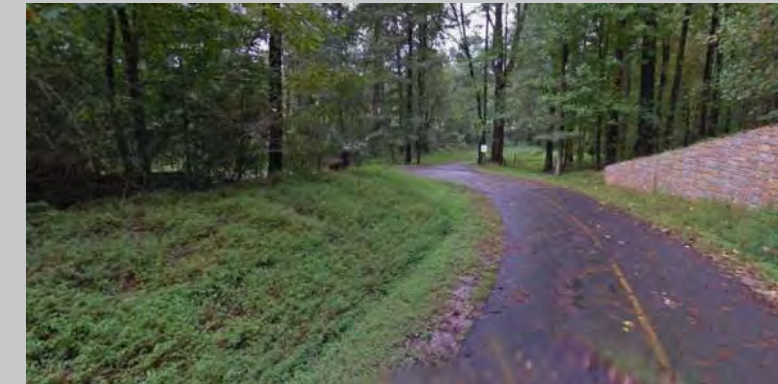
Figure 9. Limited sight lines (Source: Google Maps)
