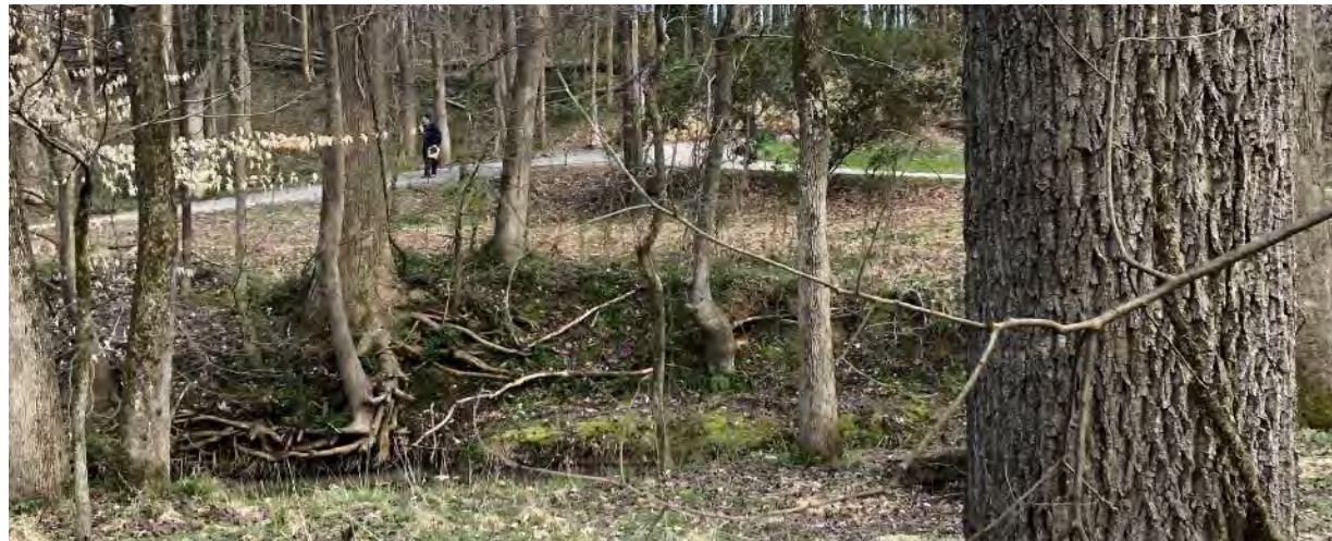
Existing oak trees near confluence, damaged by erosion
