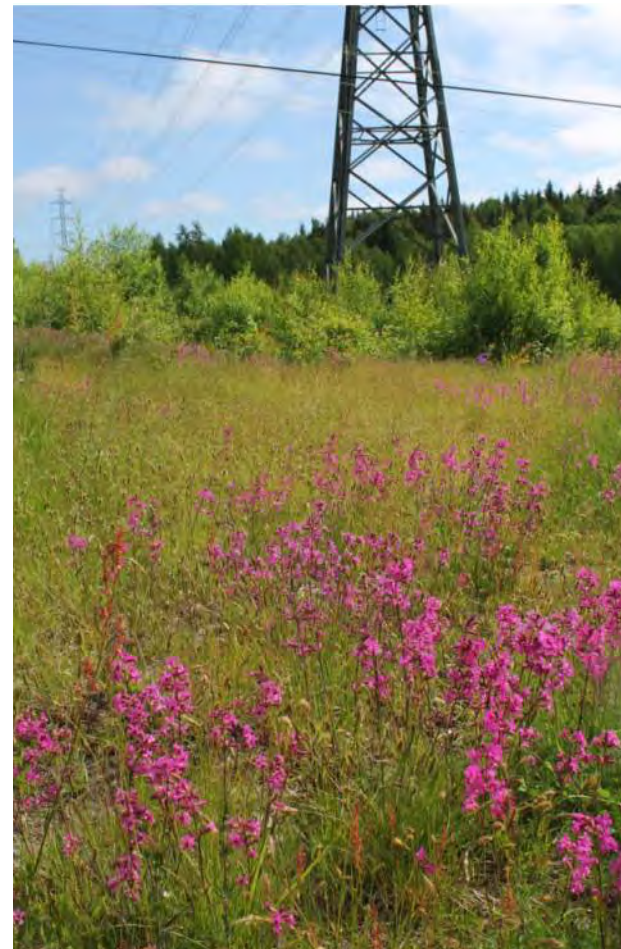
Meadow planting within power line easement, Finland; Photo: Jussi Lampinen, Kalle Ruokolainen, Ari-Pekka Huhta
