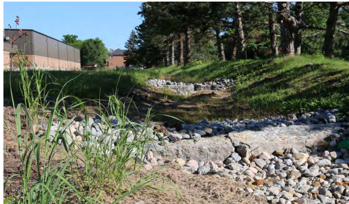
Example of proposed enhancements to swales along paths; Photo: Sustainable Technologies Evaluation Program's LID SWM Planning and Design Guide
