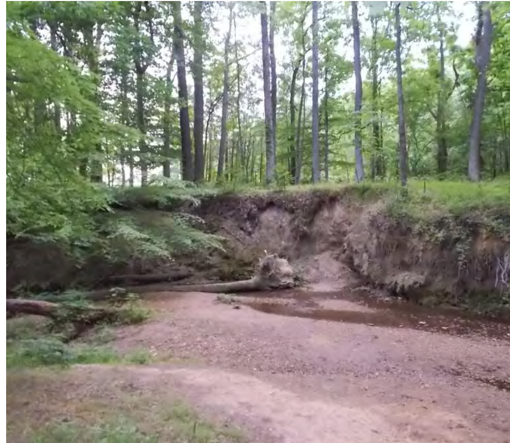
Tree loss due to erosion of stream banks (May)
