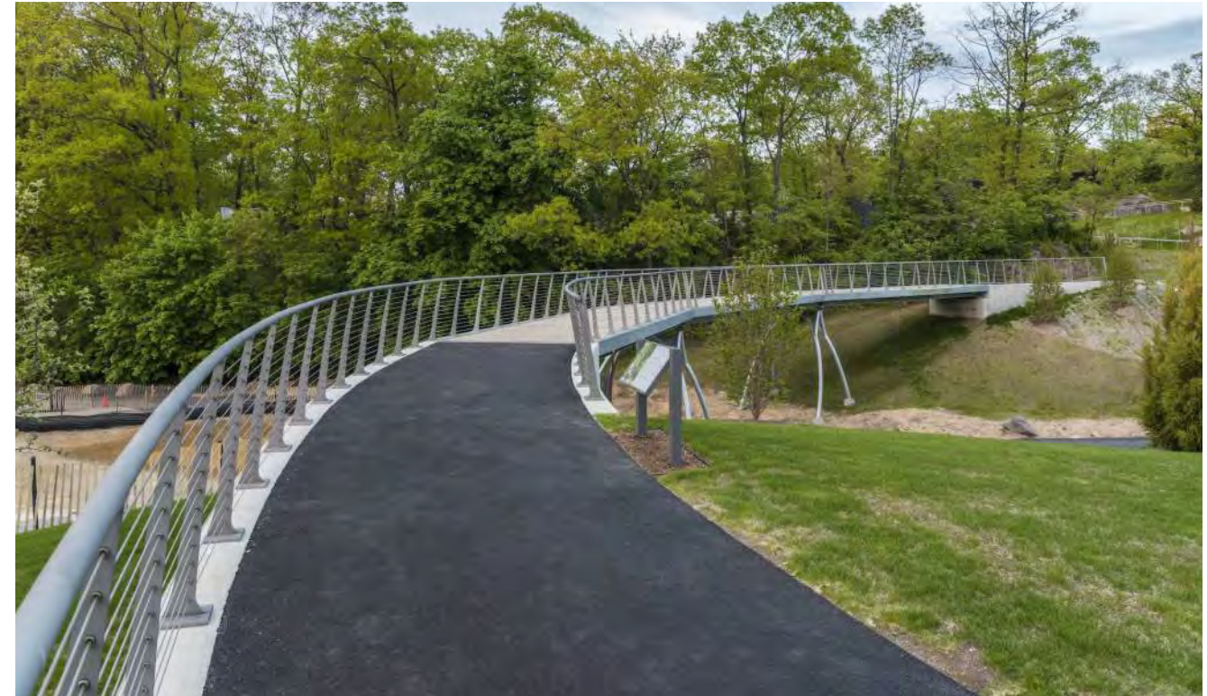
Curved span and full floodplain clearance; New York Botanical Gardens; Photo: Synergi
