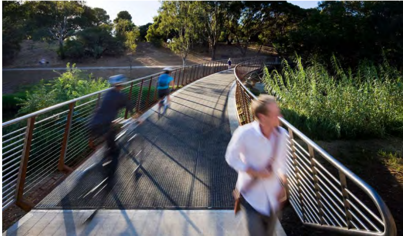
Pervious metal grating and curved span, Torrens Bridge, Australia; Photo: Sam Noonan
