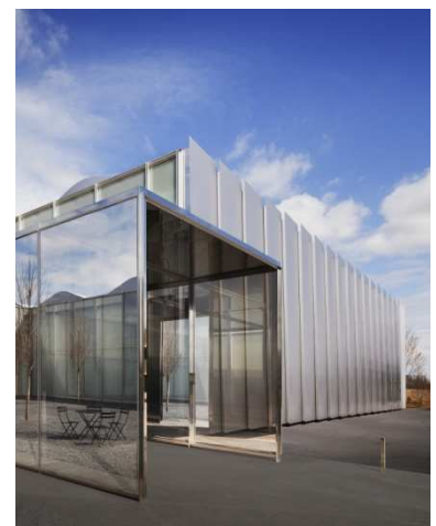
Detail, Entry Canopy. Photo by Scott Frances. Courtesy NCMA.
